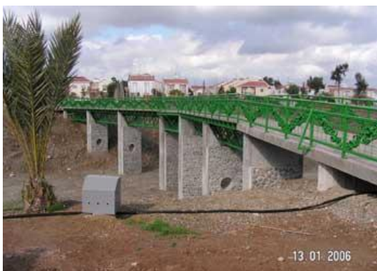
Figure 19 Bridge in Pedieos River
